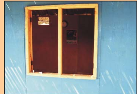
Image 48: New structure housing formerly displaced family of three, Keti Bunder Town, 5.11.07.
