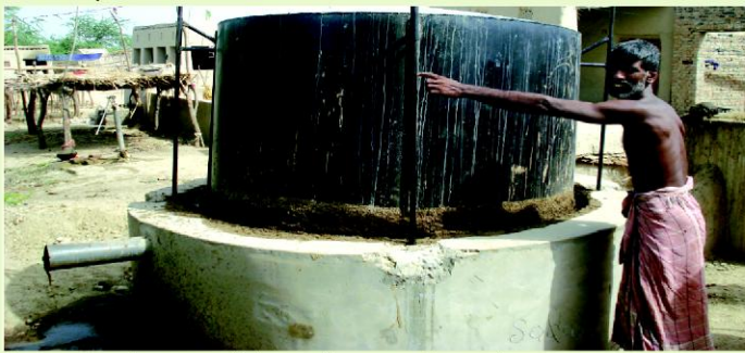
Biogas unit is being installed at a village near Chotiari Reservoir
