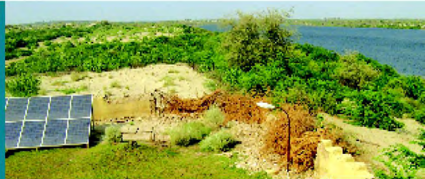
Broken boundary wall of Chotiari conservation and information centre
